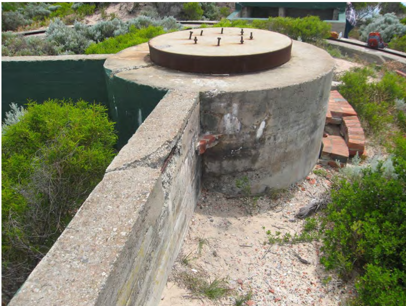
Figure 101: Gun Emplacement - rusted steel reinforcements causing chunks of concrete to blow and break off
