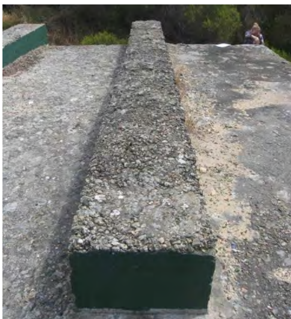
Figure 82: Operations Bunker – Reinforced concrete roof beam
