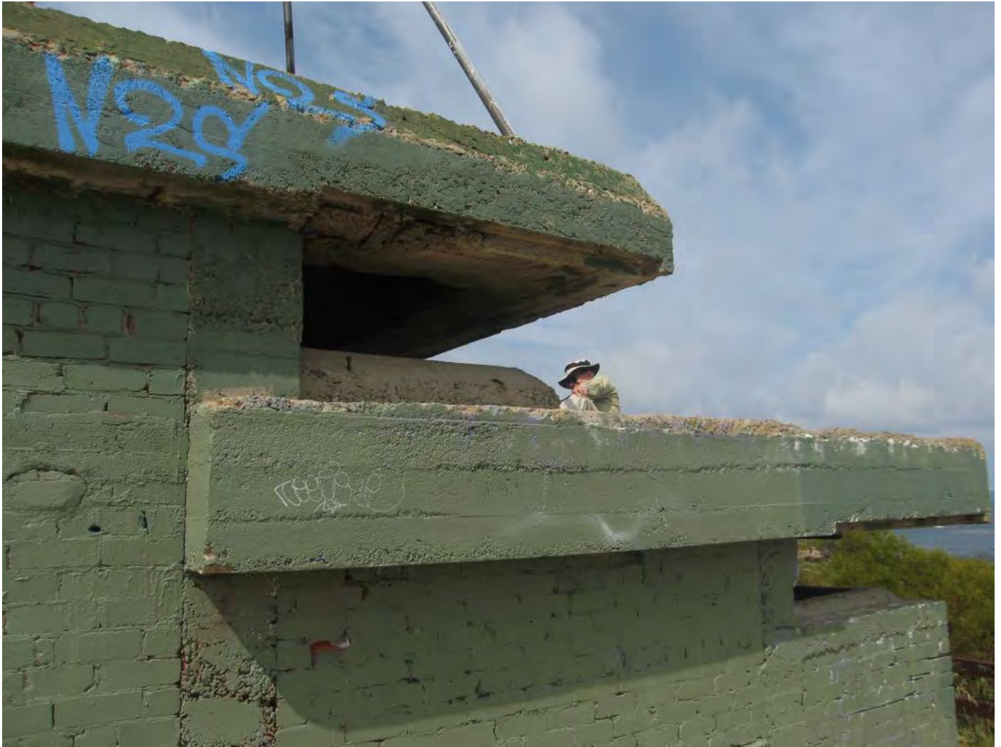
Figure 65: North Elevation – concrete overhang to the roofs providing protection to the observation openings
