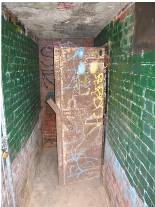
Figure 89: Operations Bunker – Extant steel entrance doors
