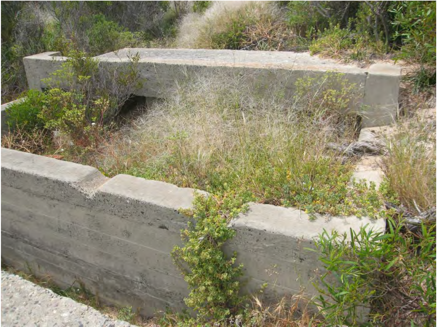
Figure 112: Gun Emplacement - Ammunition Store No. 2, sand in fill with vegetation growth
