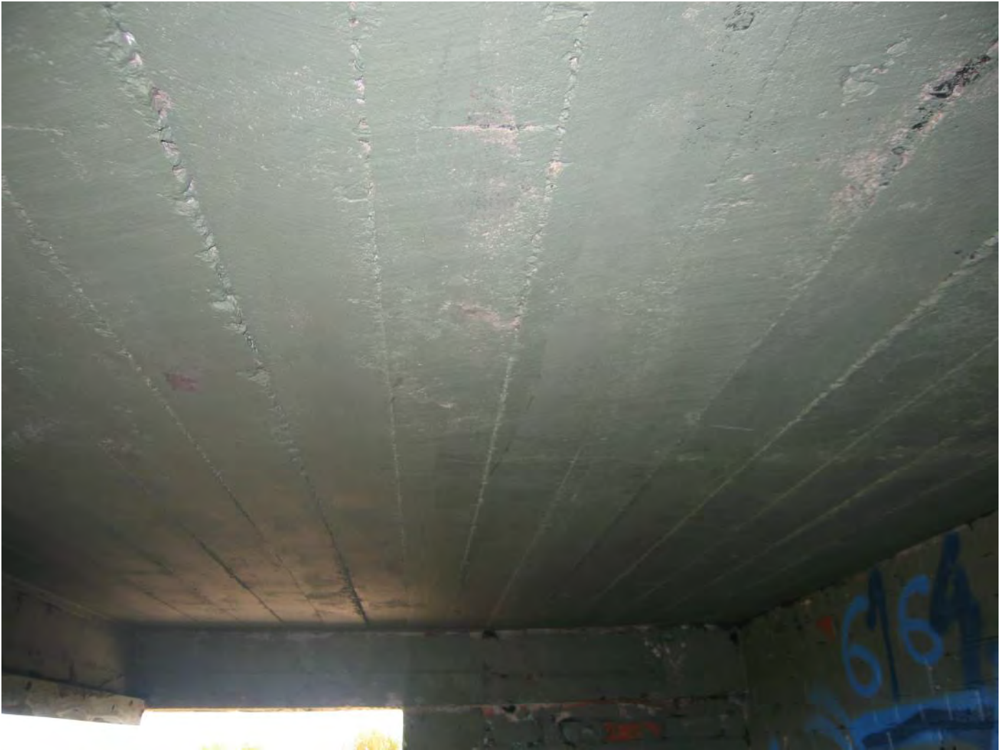
Figure 74: Concrete slab roof
