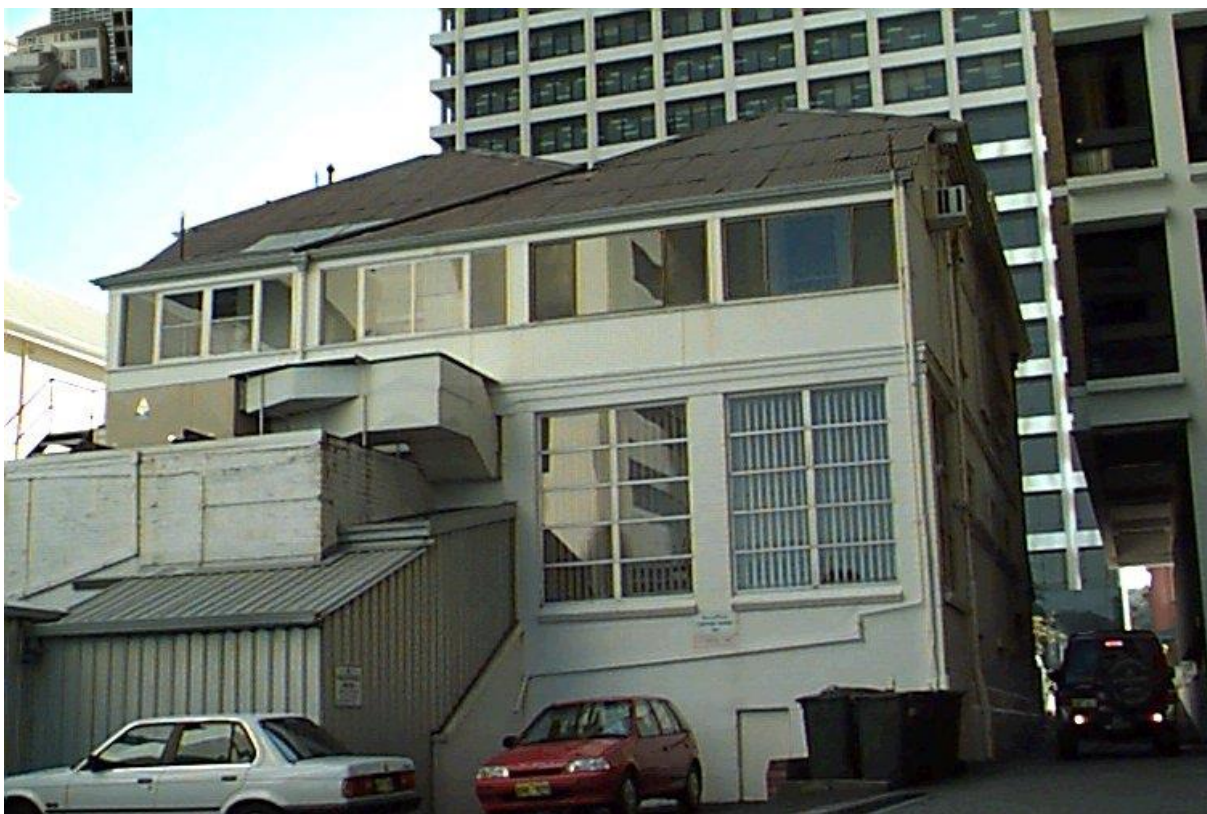
Figure 2 Northern Elevation October 1998
