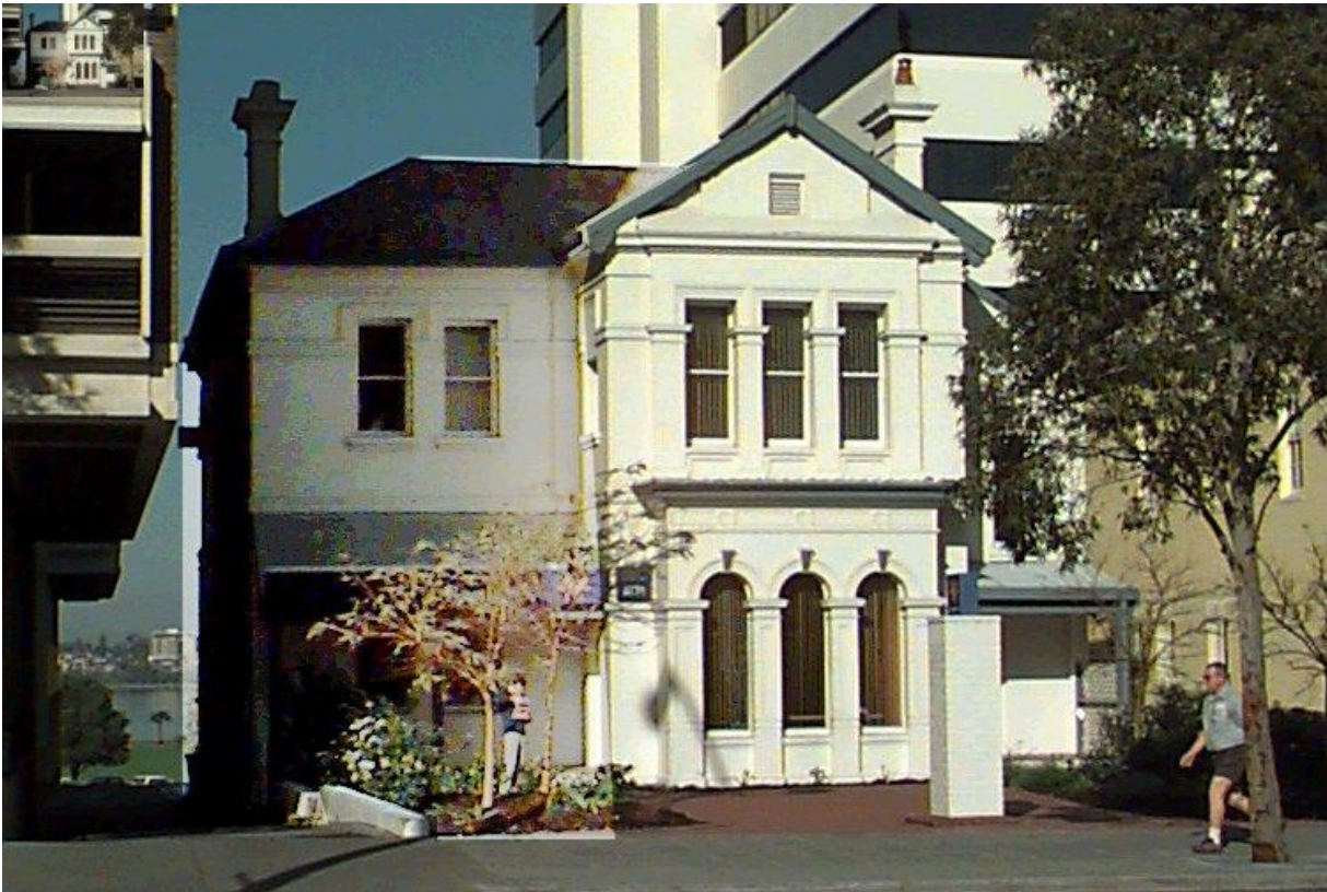
Figure 1 – Northern Elevation October 1998
